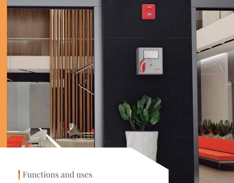
Its main purpose is the activation of the Tecnitex mobile curtain systems in the case of fire, controlling the status of the systems in real time, reporting and keeping a record of events or anomalies during the lifespan of the system.
